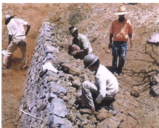
Photo: Terrace construction for erosion prevention, Isle of Fogo, Cape Verde.
