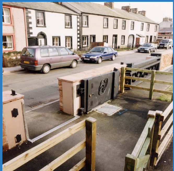
Flood gate to protect properties against flooding.
